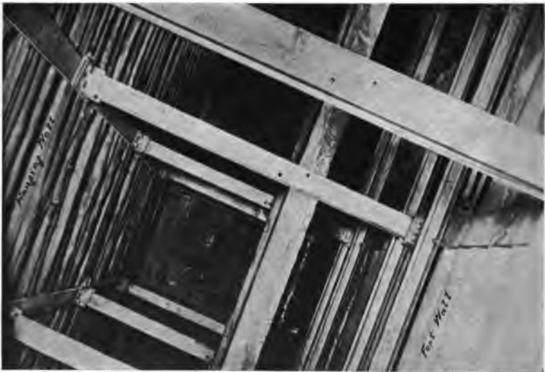
Fig. 17. Steel Framed Shaft, Newport Mining Co., Ironwood, Mich.
